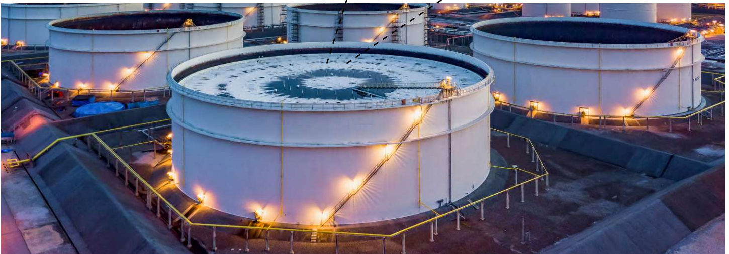
Fuel Storage Floating Roof Top Tank
